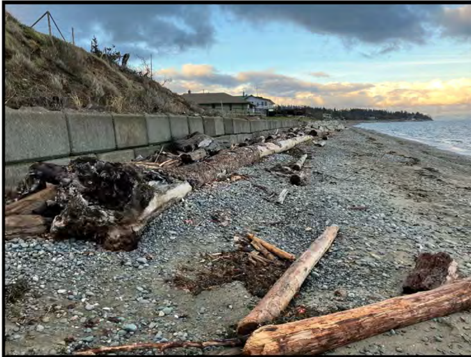
Photo 3.2 - View of property foreshore conditions, facing northeast
