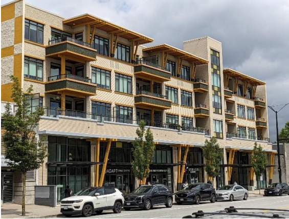
Figure 15: The primary pedestrian entrance to commercial units at grade should be from the fronting street (Guideline 5).
