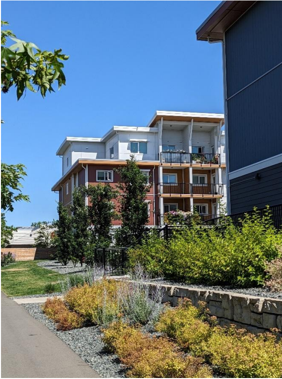
Figure 13: Break up the building mass by incorporating design elements that clearly define the base, middle, and top of the structure (Guideline 38). Private balconies should consider sightlines into adjacent properties and consider step backs to reduce visual and shadow impact on neighbours (Guideline 43).
