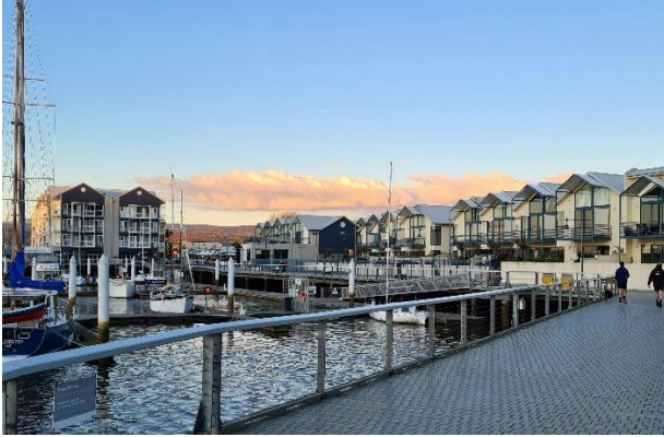
Figure 20: Building character should be commercial or residential in nature and not industrial or utilitarian (Guideline 65).
