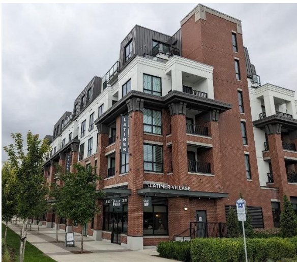
Figure 18: Upper storey step backs; variety of colours, roof lines, building materials and architectural features that reduce perceived height and massing (Guidelines 38-39). Flat panel siding used as accent on building rather than dominant material, and seams blend in due to use of flashing that is same colour as panels (Guideline 43).
