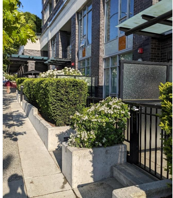
Figure 14: Residential units at grade should have transitional areas between the building façade and public circulation with landscape screens (Guideline 4).
