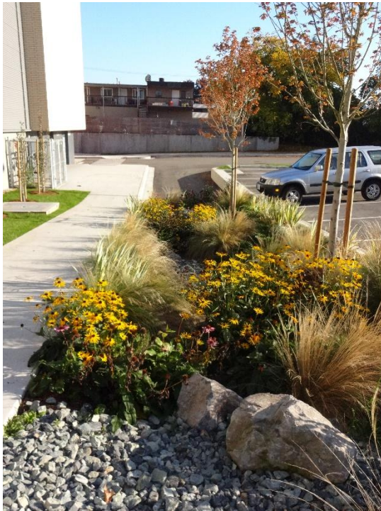
Figure 24: Landscaped areas with the capacity to infiltrate and accommodate stormwater, such as planting beds and rain gardens, are encouraged to reduce stormwater runoff from surface parking lots and rooftops (Guideline 23).
