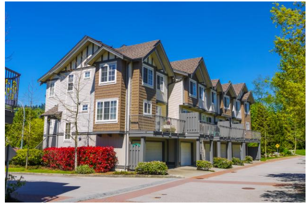
Figure 10: Use a variety of colours, rooflines, architectural features and building materials to create interesting façade treatments (Guideline 35).
