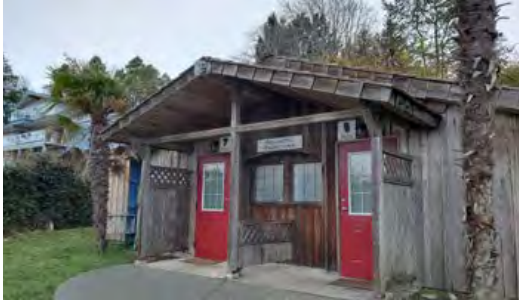
Existing: Washroom at Filberg Heritage Park
