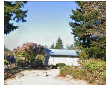
Existing: Washroom at Aspen Park
