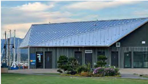
Existing: Washroom at Marina Park
