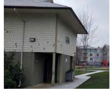
Existing: Washroom at Anderton Park
