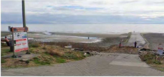
Existing: Point Holmes boat launch
