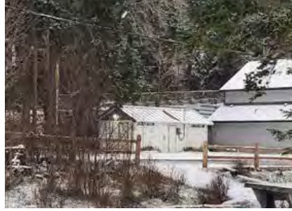
Existing: Washroom at Kye Bay
