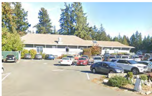
Existing: The parking lot and clubhouse are the main entry to the site from the Downtown interface (across from Comox Mall).
