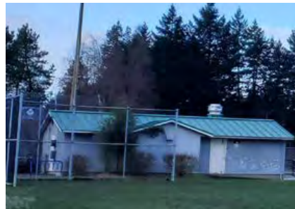
Existing: Washroom at Highland Park
