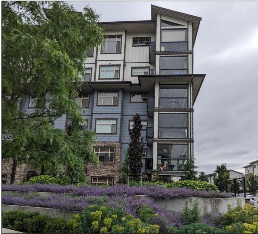
Figure 4: This six-storey residential building does not have step-backs but utilizes other landscaping and architectural techniques that contribute to reducing the perceived height and massing, including material / colour variation, a cornice/overhang detail at the fourth storey, and tiered landscaping features and sufficient landscaping space to accommodate a large shade tree.
