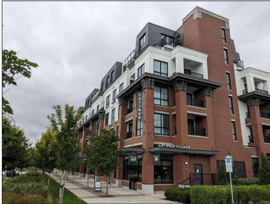
Figure 3: Figure 18 in Development Permit Area 4 – Commercial and Mixed Use. This is a six-storey mixed-use building with step-backs at the fifth and sixth storeys. In addition to step-backs, the building utilizes material variation, weather-protection overhangs, and cornice line details at the third and fourth storeys. All these features contribute to reducing the perceived height and massing of the building.
