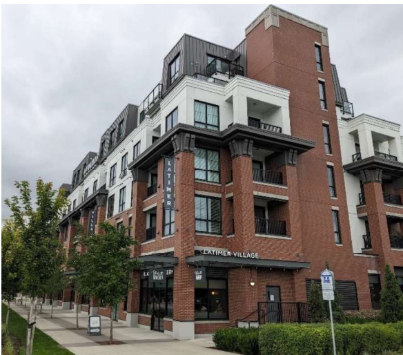
Figure 18: Upper storey step backs; variety of colours, roof lines, building materials and architectural features that reduce perceived height and massing (Guidelines 38-39). Flat panel siding used as accent on building rather than dominant material, and seams blend in due to use of flashing that is same colour as panels (Guideline 43).
