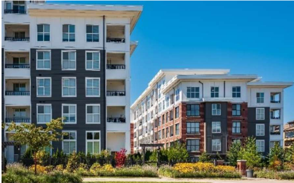
Figure 13: Break up the building mass by incorporating design elements that clearly define the base, middle, and top of the structure (Guideline 38). Use higher quality (smaller scale, fine grained) materials at the pedestrian level (Guideline 40). Private balconies should consider sightlines into adjacent properties and consider step backs to reduce visual and shadow impact on neighbours (Guideline 43).
