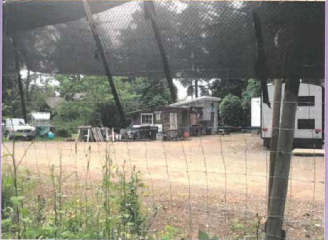
*Unightly and *over 35m' outbuildings *over 6 meters wide dust parking (contrary to bylaws) ** ① ② ③ ④ coach house screening
