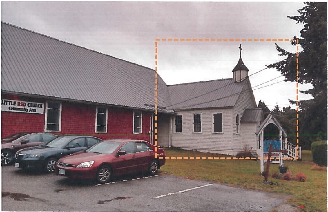
Subject structure in October 2019 with metal roof
