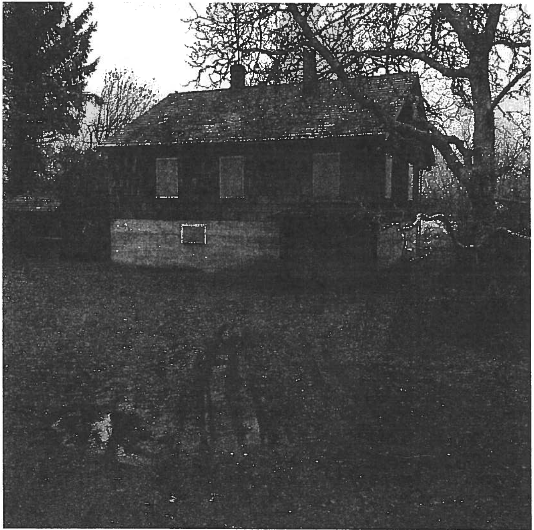
Jan 17 th 2016. The approaches are wet and unstable.
