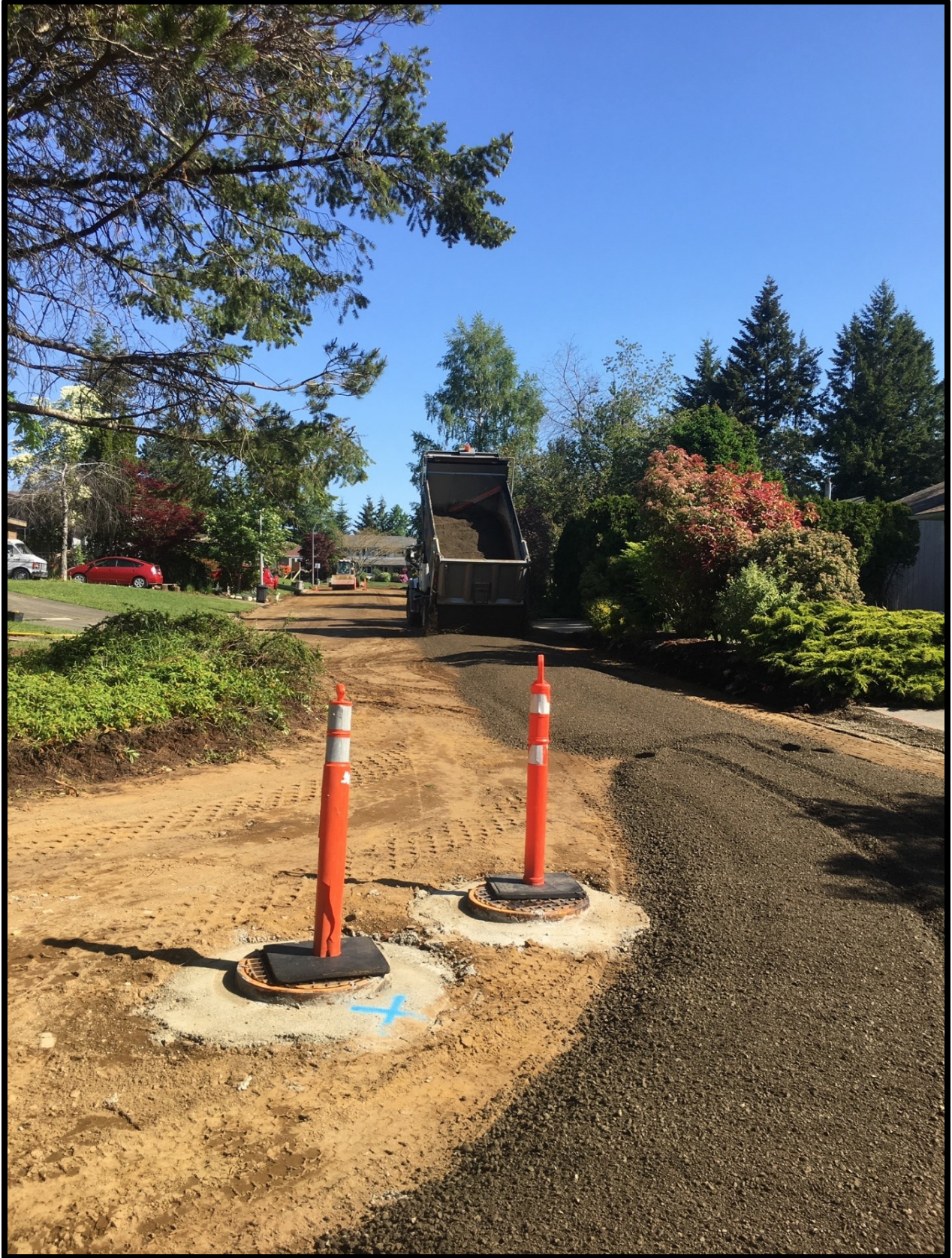
New road surface on Bambrick Place
