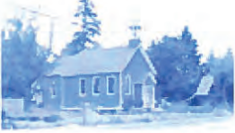
3: St. John the Baptist Church: built 1885, rebuilt 1889
