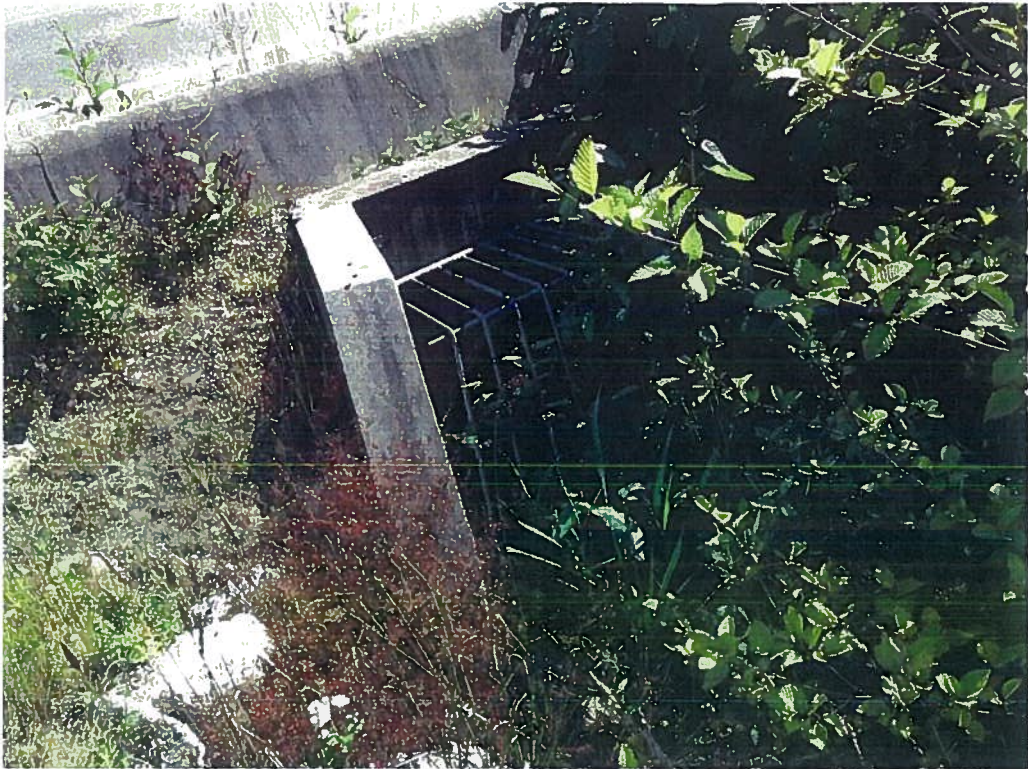
Photo #41 – Culvert Headwall (crossing Knight Road west of Airport)
