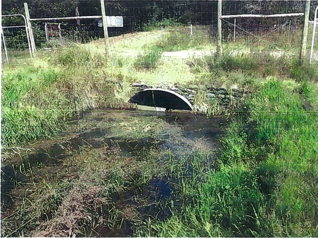
Photo #37 – Rudimentary control structure near outlet of Queen's Ditch
