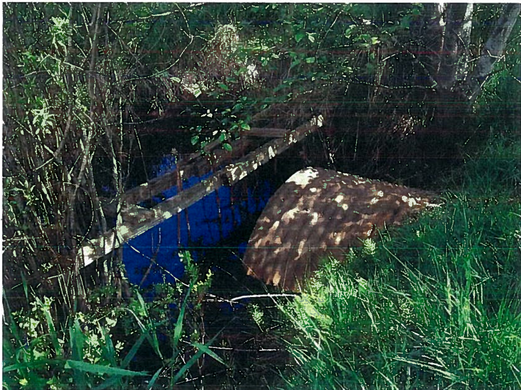
Photo #30 – Farm Ditch culvert outlet with abandoned outlet control
