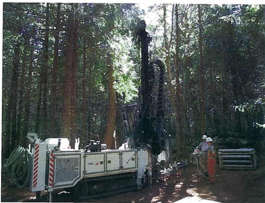
Photo 1: Boart Longyear Mini-Sonic drill drilling a borehole at the Site
