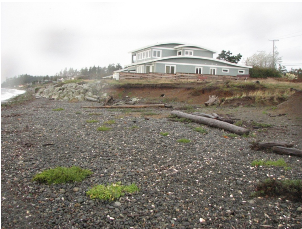
Photo 4 (4086): Top of berm el. = 4.5m; top of riprap el. = 3.5m; ocean level = 1.3m CGD
