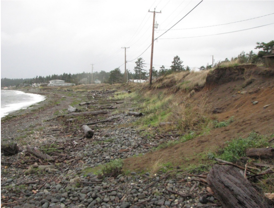
Photo 3 (4087): Top of berm el. = 5.4m; base of slope el. = 3.0m; ocean level = 1.3m CGD
