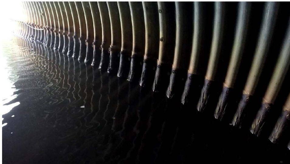
Photo 4 Varied Corrosion, Light to Very Severe at Water Line [Inlet, Looking Upstream, River Left]
