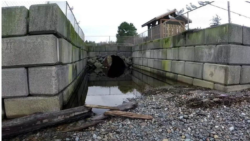
Photo 11 Outlet Channel & Debris Blocking Flow Path [Looking Upstream]
