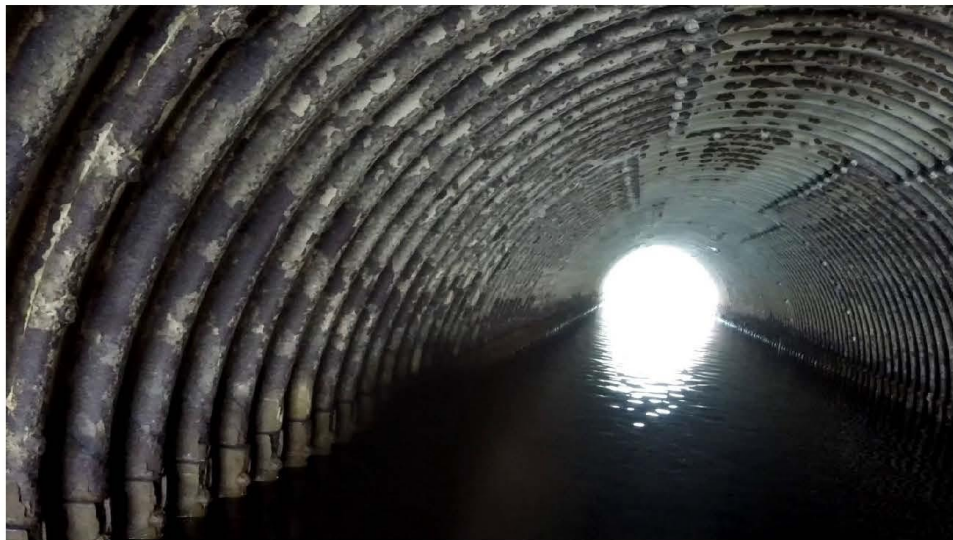
Photo 6 Moderate to Very Severe Corrosion [Outlet, Looking Upstream, River Right]
