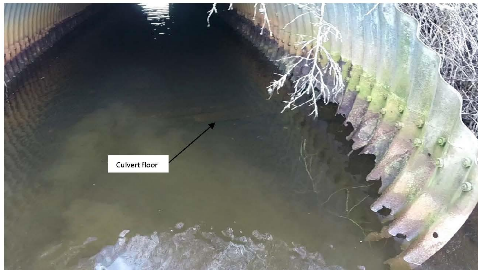
Photo 3 Missing Pipe Floor [Inlet, Looking Downstream]
