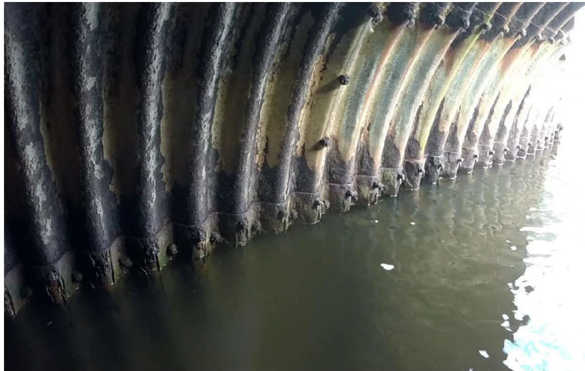
Photo 5 Moderate to Very Severe Corrosion [Outlet, Looking Downstream, River Left]
