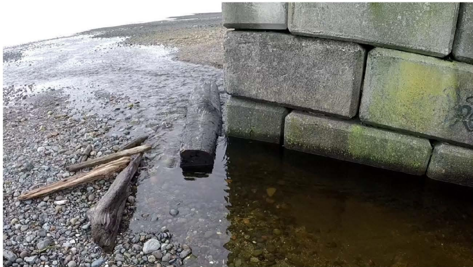
Photo 13 Undermining Retaining Wall [River Right, Looking SE]
