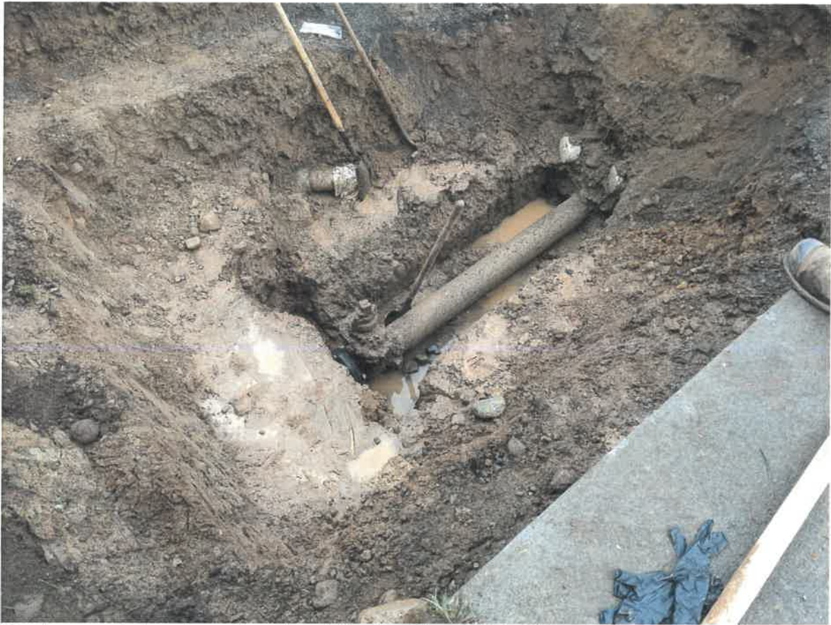
Replacement of watermain valve at Nootka St and Tsimshian Ave
