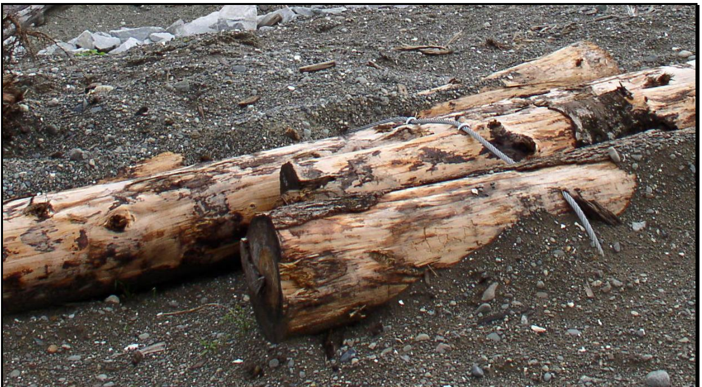
Some of the anchored logs in the Lazo Road restoration project
