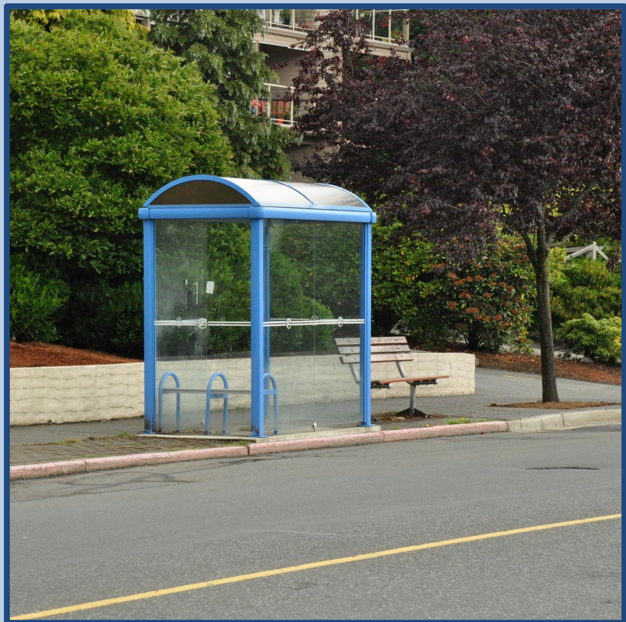
New bus shelter – Comox Avenue at Ellis Street
