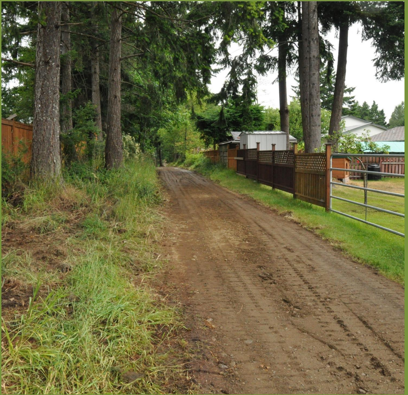
Construction of the Cottonwood Greenway – to be completed in 2013
