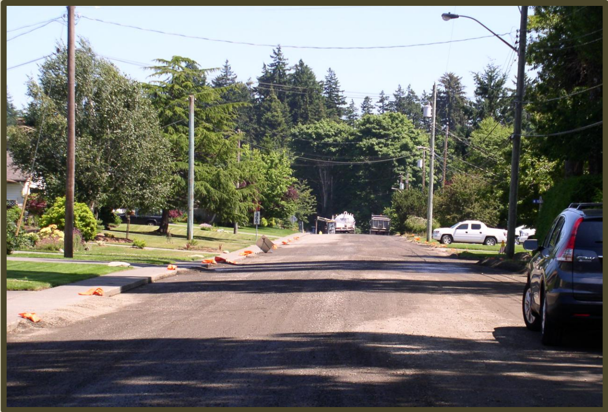
Comox Avenue east of Pritchard Road, in preparation for repaving
