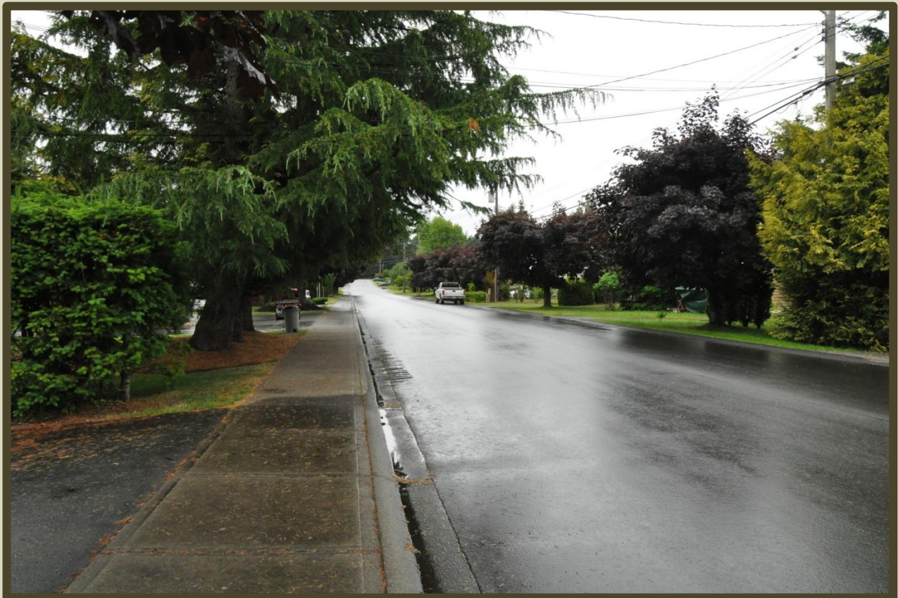
Dogwood Avenue repaved
